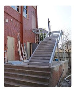
The Capital works on Presentation Campus to replace the dilapidated Emergency Exit Stairs on the Rahilly Building are nearing completion. The old wooden stairs are being replaced with new galvanised steel stairs that will make the exit route from the first floor of the building safe for students and staff should an emergency occur in the future.
